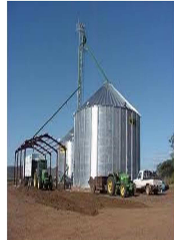
Modern silos under construction
